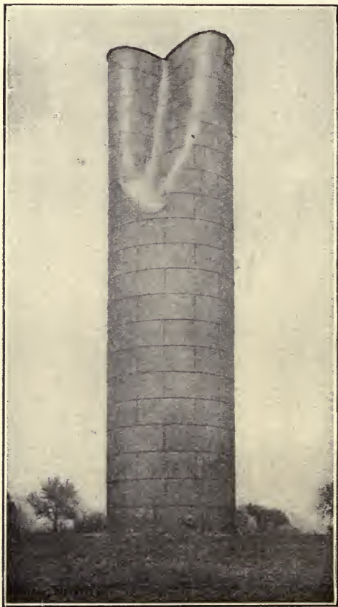
FIG. 7.—VIEW SHOWING EFFECT OF WIND ON STAND-PIPE AT LINCOLN, NEB. ( Engineering News. )
